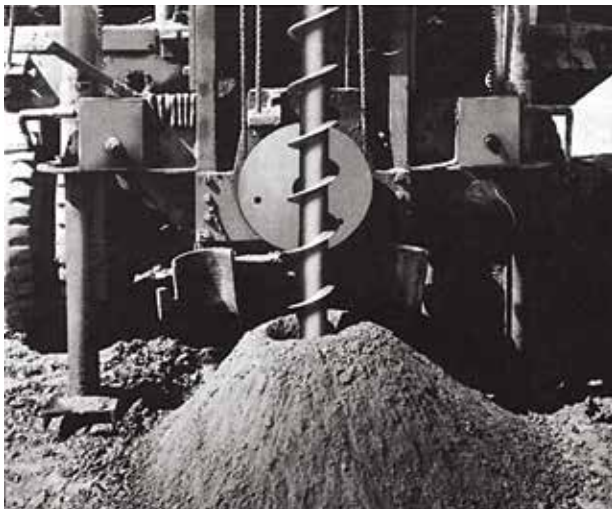
Auger with BD Head drills blast hole.
