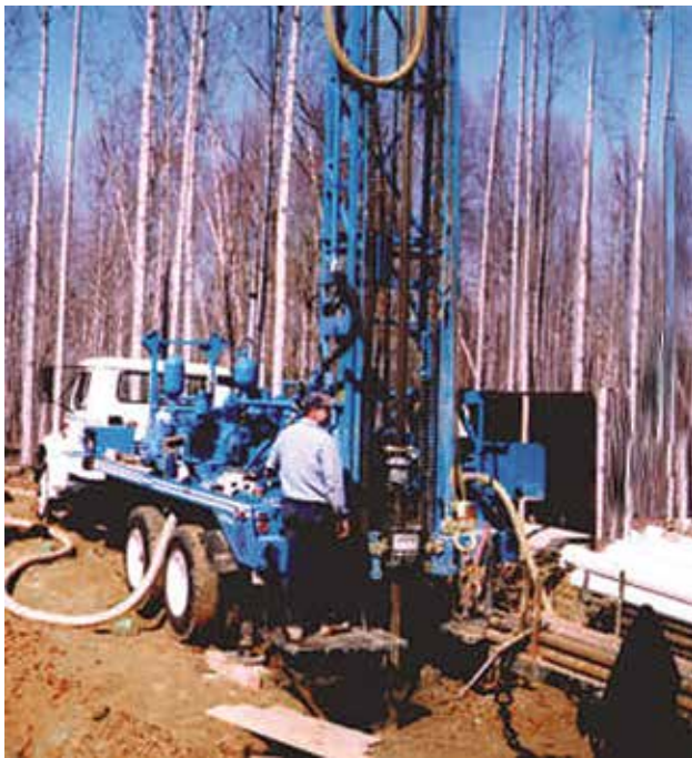
Drilling water well with Blue Demon BDA Drill Head.
